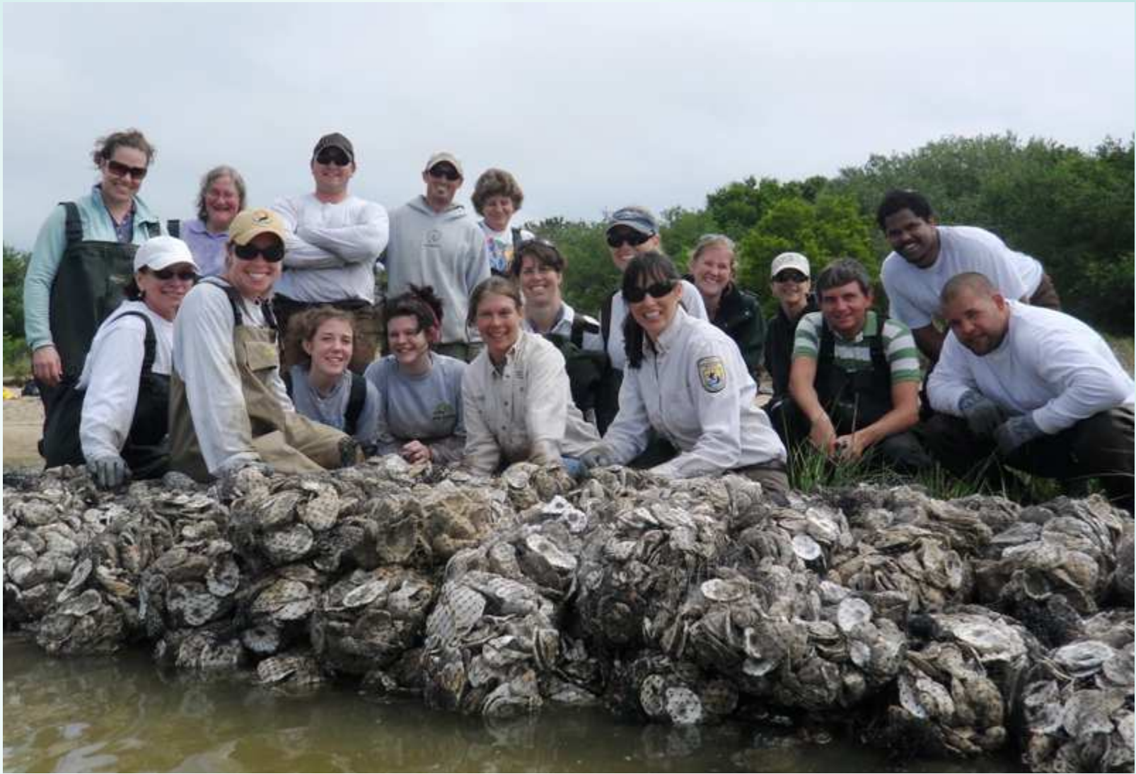
Volunteers construct a sill at Jockey's Ridge State Park
